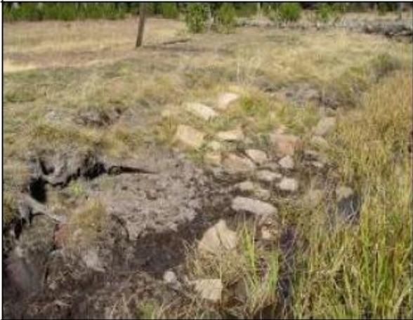
Lower reach, eroded & trampled banks, failed gabion.
